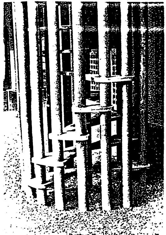
Detail of external staircase in tall building of la Muette district in Drancy
